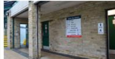
Existing Halifax bus station public toilet
